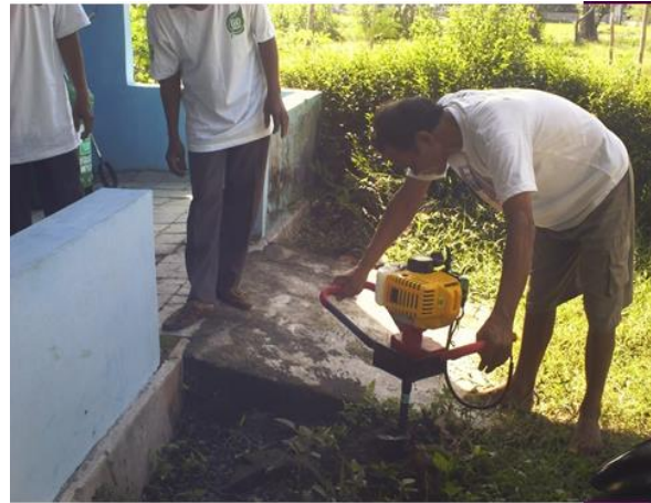
Gambar 7: Pengeboran Lubang Resapan Biopori (LRB)
